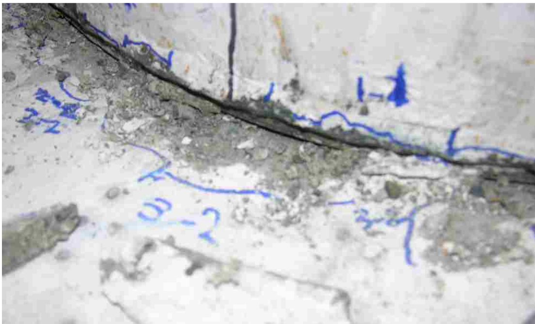
Figure C.10 Footing fillet-spalling.
