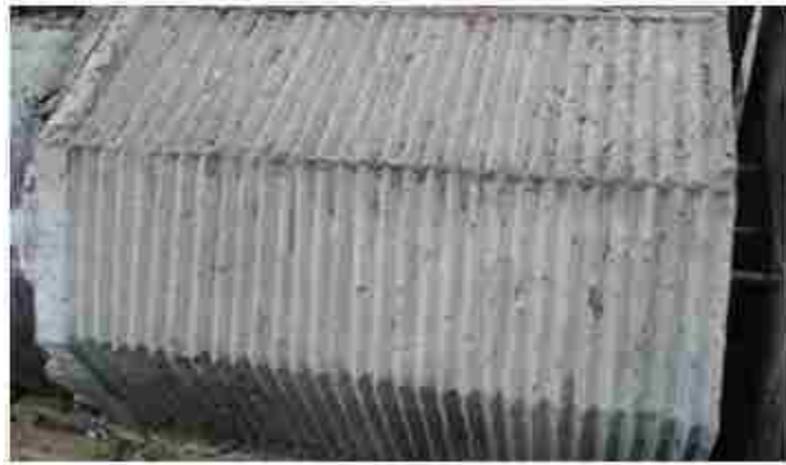
Figure 2.10 Roughened surface of the portion of the column that extends into the spread footing.
